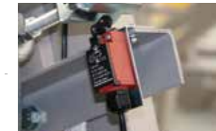
Step chain loosen and broken protection
